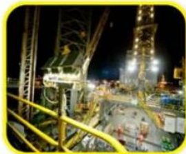
Petrol Process Factory
