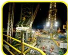
Petrol Process Factory
