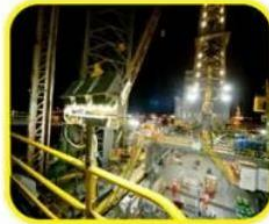
Petrol Process Factory
