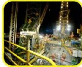
Petrol Process Factory
