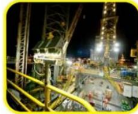
Petrol Process Factory
