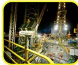
Petrol Process Factory
