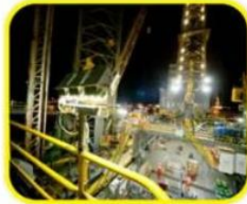
Petrol Process Factory
