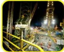
Petrol Process Factory
