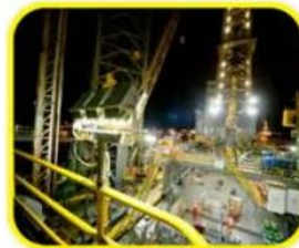
Petrol Process Factory
